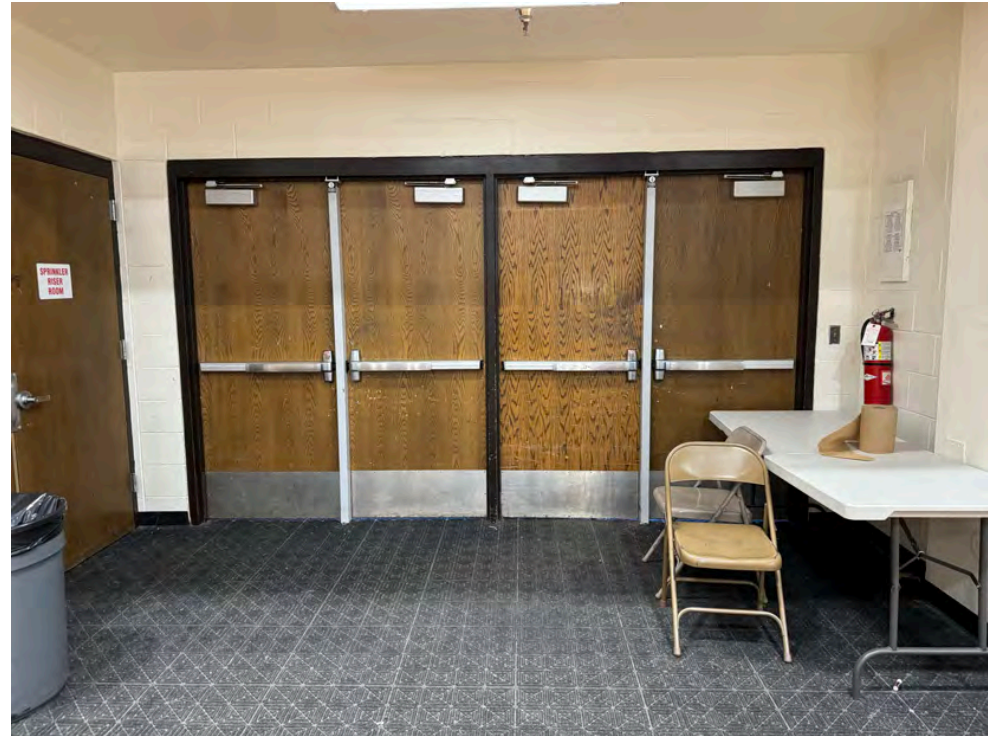
Unit Exit from Floor Folding 6' 8" tall 5' 10" wide
